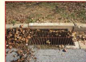
1 Storm water containing sediments, motor oil, fertilizers and other surface pollutants from the roads, residential industrial and commercial properties wash into the municipal storm system through the storm drains.
