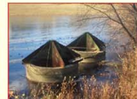
3 Riser Pipes discharge water from the retention pond after sediments and heavier pollutants settle to the bottom.
