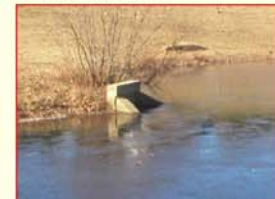
2 Storm water enters retention pond through this endwall.
